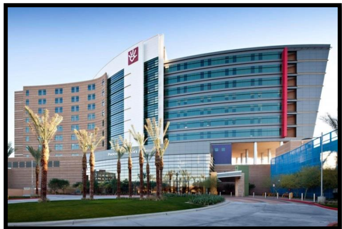
Figure 17:: la façade de l'hôpital PHENIX.source:archdaily.com
