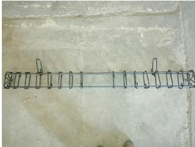
Figure II.11: Ferrailage des poutres.
