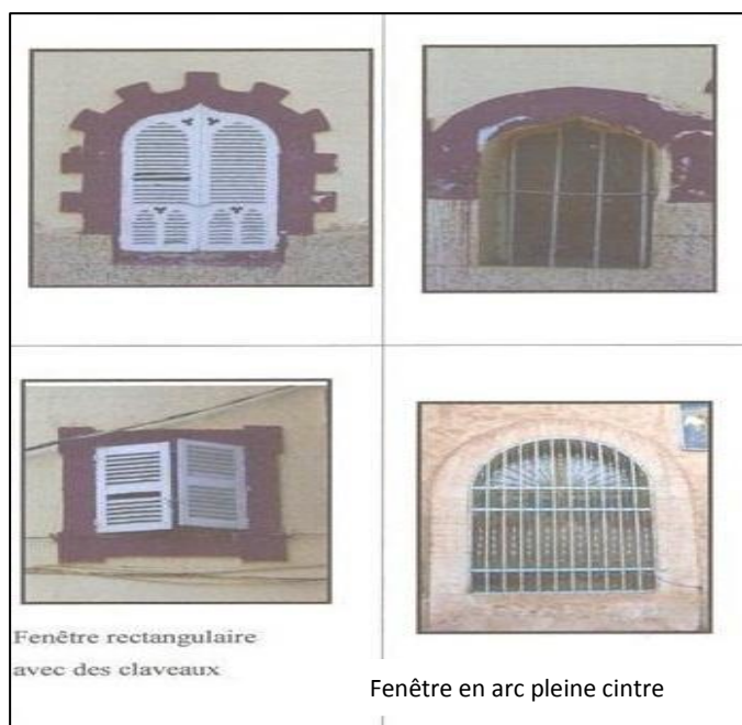
figureII.35 :LES FENETRES SOURCE : THESE REHALIBITATION DES ESPACES PUBLICS (BOUDELAA
