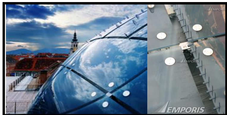
Figure.I.32 :revetment de musée ,Source : https://www.emporis.com/buildings/236175/
