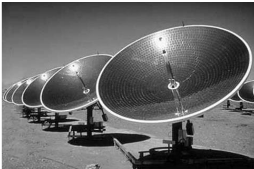
Figure I. 6. Parabolic dish concentrating solar power (CSP) systems [21]
