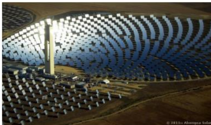
Figure I. 11. View of the PS20 power plant (source: Abengoa Solar) [22].
