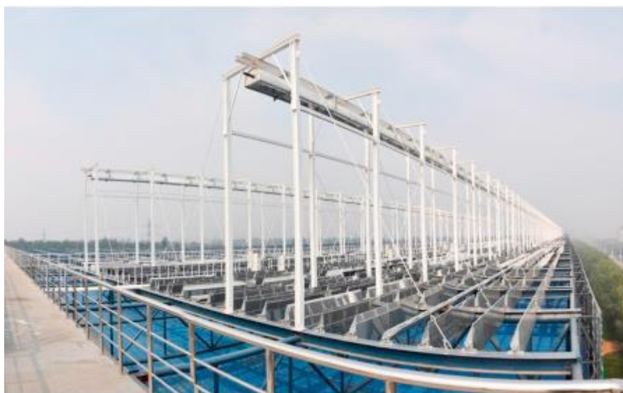
Figure I. 4. Linear Fresnel reflector solar power generation [19].
