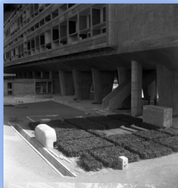
Figure 77: l'accès secondaire 1945-1979 Source : https://www.flickr.com/photos/reconstruction1945-1979
