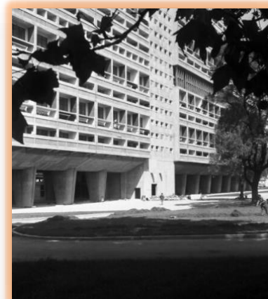
Figure 79: l'accès principale 1945 Source : https://www.flickr.com/photos/reconstruction1945-1979
