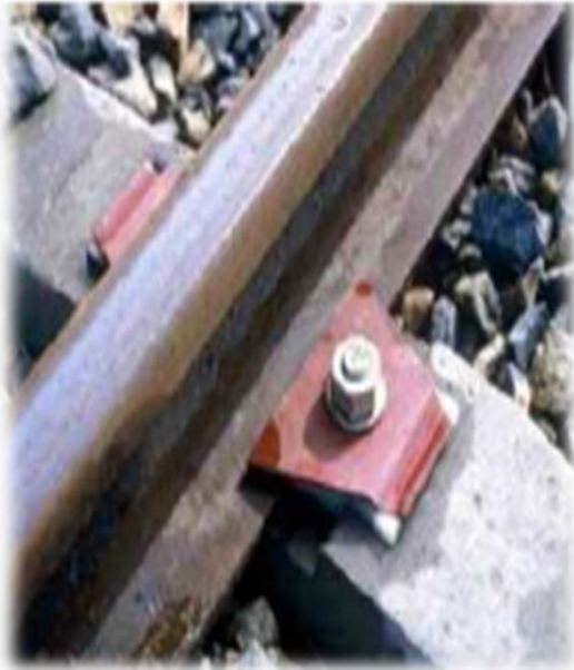
Figure IV.16 : attache de type Nabla
