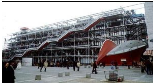
Figure N 28 : Pompidou, France.
