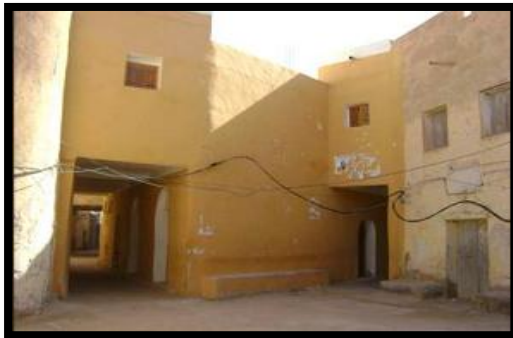
Figure I.11: Aménagement placette, ksar Ouargla
