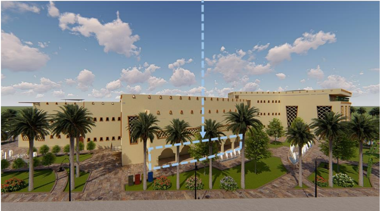
Figure 150: la façade Nord
