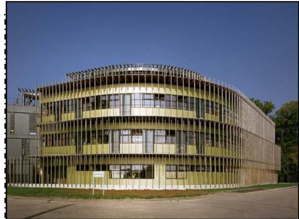
Fig.II-28 façade sud Source : Source : [http://www.whrc.org/building/pdf/Building]
