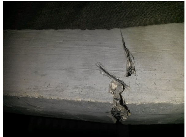
Figure III.6- Couture des fissures
