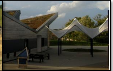
Figure 40 : structure textile Source : http://www.bhpp.co.uk
