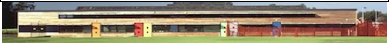
Figure 64 :façade sud Source : timothysoararchive.co.uk
