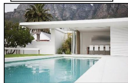
Figure 15 :toiture plat Source : www.terrain-construction.com
