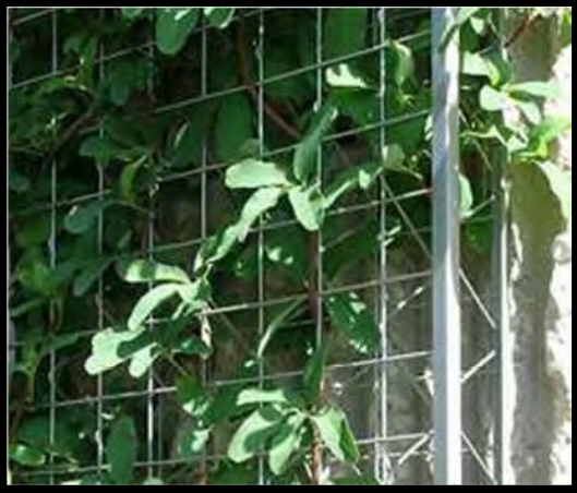
شكل 4-20- وحدات التعريشة القياسية المصدر: Sam C. M. Hui, Benefits and potential of vertical greening systems, 2011, Department of Mechanical Engineering, The University of Hong
