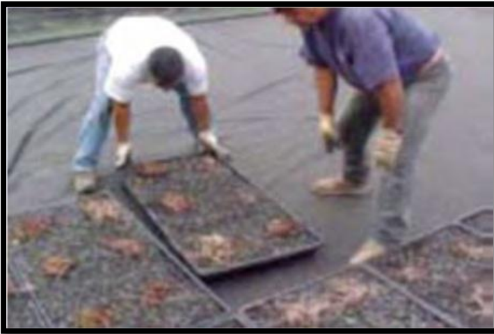
شكل 4- 15 - نظام تركيب الوحدات المصدر: Annika McIntosh, Green Roofs in Seattle, a survey of vegetated roofs and rooftop gardens, the University of Washington, September 2010
