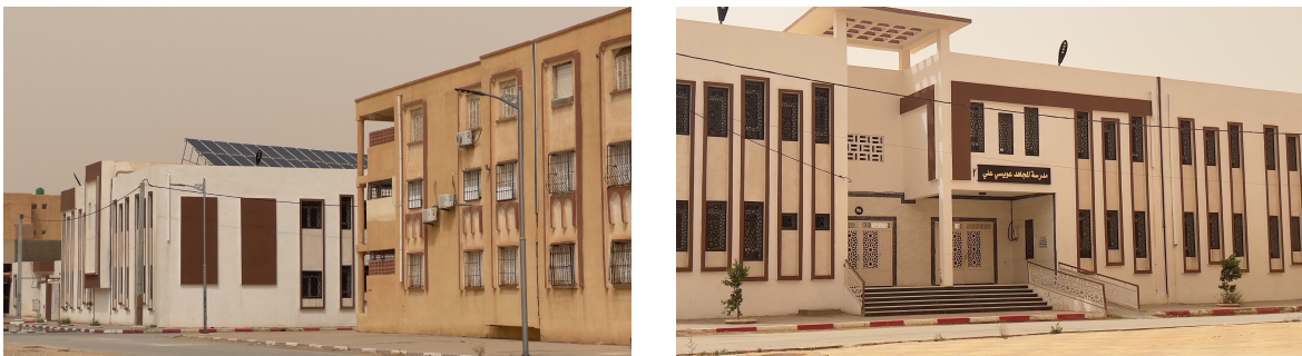
Electrification by photovoltaic system of Aouissi Ali primary school, Laghouat.
