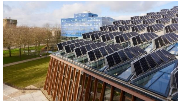
Figure 272 : Panneaux photovoltaïques Dynamic. Source: www.arch.daily.com.
