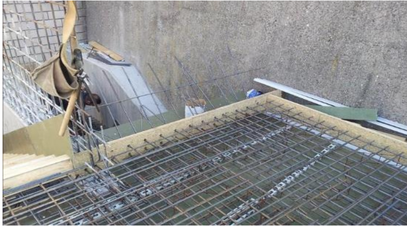
Figure 3.8. Ferrailage de pallier.
