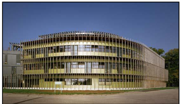
Fig.II-28 façade sud Source : Source : [ http://www.whrc.org/building/pdf/Building ]
