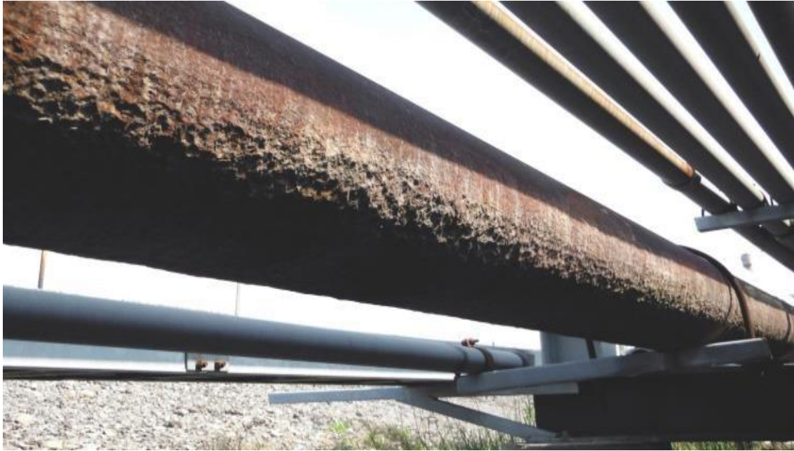
Figure 2.1: Corrosion Externe
