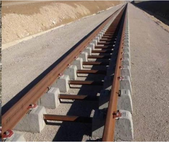
Figure I.16 : Traverse Bi bloc.
