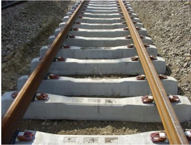
Figure I.15 : Traverse Monobloc.
