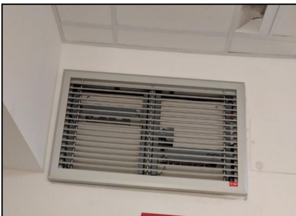
Figure 228 volet coup feu https://www.cmsi-securite.com/desenfumagemecanique.php
