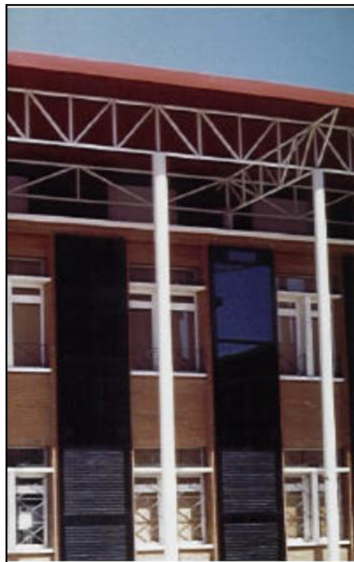
Figure 85: La façade sud
