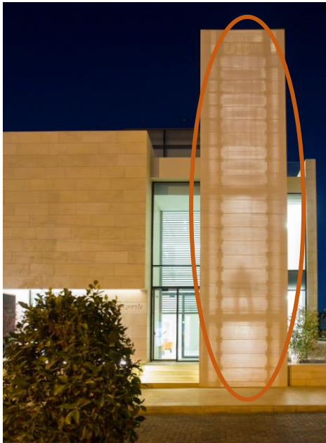
Figure 35 transparence de la façade Source: archdaily
