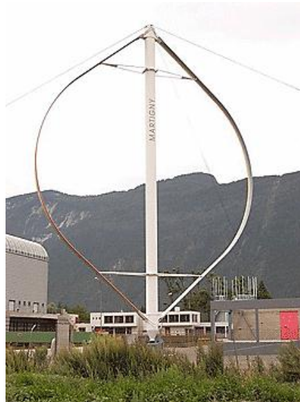
Fig.I.8. Darrieus vertical-axis wind turbine in Martigny, Switzerland
