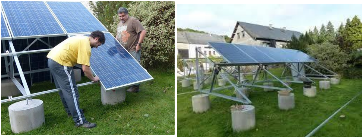
Figure II.2: Montage des supports des modules
