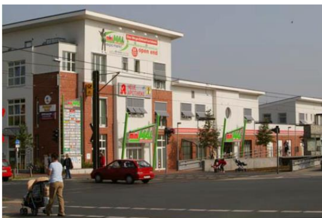
Centre commercial et de services
