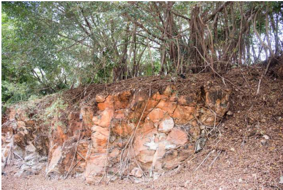
Figure.IV.4: Granite block partly eroded by plants.
