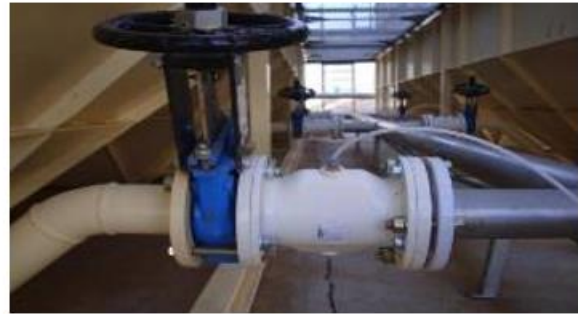
Figure IV 3: Pinch valves
