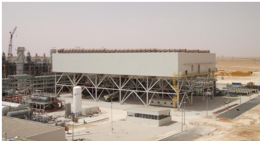
Figure IV 26: The SPX air condenser of the power plant [20]
