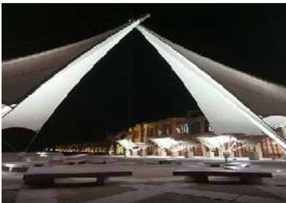
Figure I.22: photo des auvents Source: Architectural Precast Concrete Panels Beautify Facade of Kuwait Scientific Center
