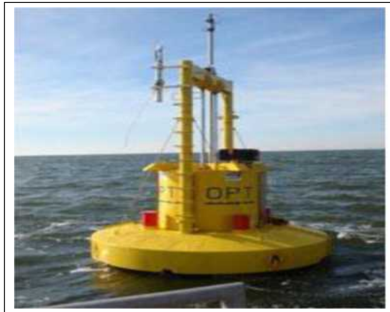
Figure (2.9): Système Power Buoy (Ocean Power Technologies)Ref: [21]
