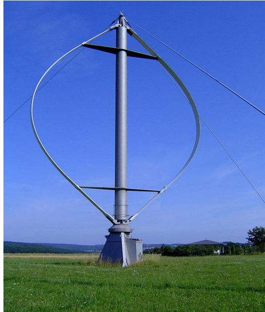
Figure 1.4 : turbine a axe vertical [9]
