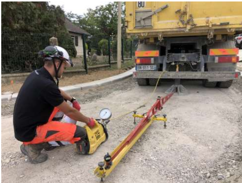
Figure II.7 : Essai de charge sur plaque
