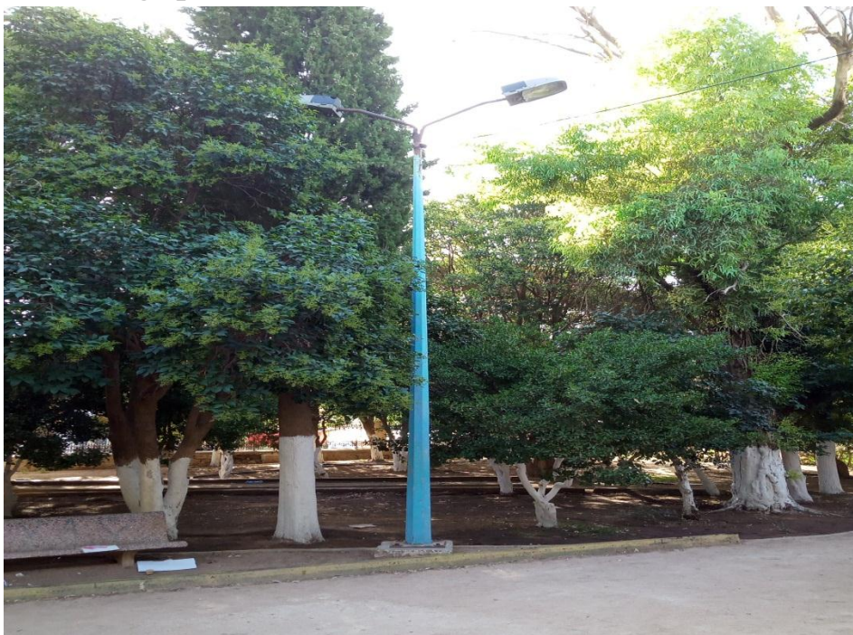
Figure n° 25: poteau d'éclairage public
