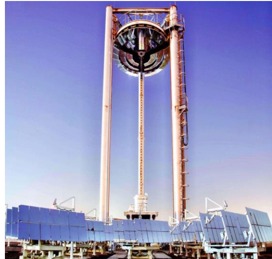
Fig.33 : la centrale solaire Masdar City (Source : https://cleantechnica.com )
