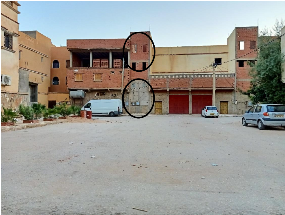
Figure III. 102 : MATERIAUX DE CONSTRUCTION (BRIQUEE ROUGE/PARPAING/CIMENT)
