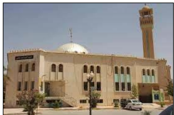
Figure III. 84 : MOSQUEE AHMED HAMANI
