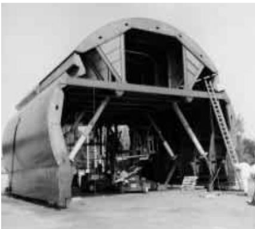
Figure IV.27 : Coffrage de tunnel [22]
