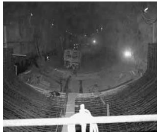
Figure IV.26 : Armatures de radier [22]
