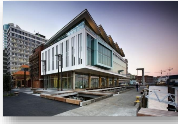
Figure II. 30:photo de Meridian office source : architectures.jidipi.com
