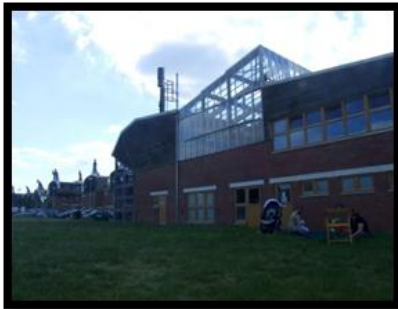
Figure III.11 : façade BDZ (la source : Google image)
