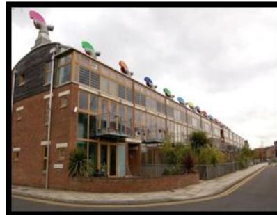
Figure III.12 : façade BDZ (la source : Google image)
