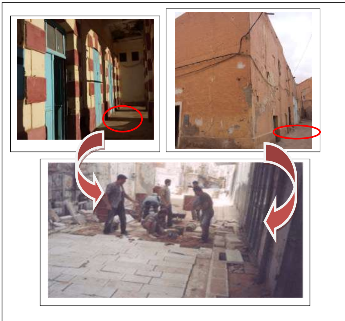
Figure 43 : Pavage des ruelles, (Source: Z.Damene, M.S.Goual, T. Bourzeg, Y.Daikh , jan 2015, Study of pathological cases in the district of Zegague Elhadjaj, Journal of fundamental and applied sciences , p 74).
