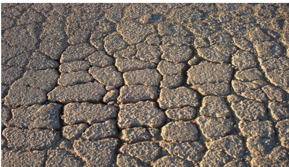
Figure II.13 : Fissures en carrelage .
