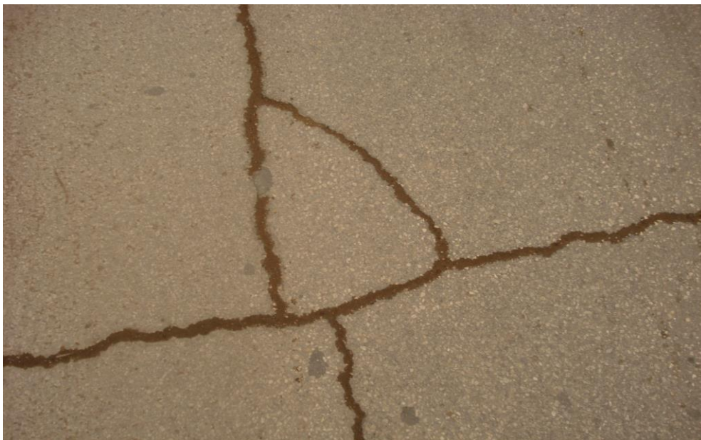
Figure II.11 : Fissures transversales .
