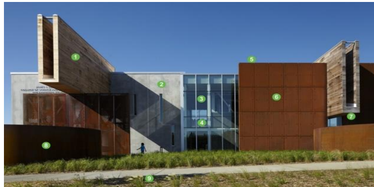
Figure 14 : Façade nord. (UMD Swenson Civil Engineering Building / Ross-Barney Architects)
