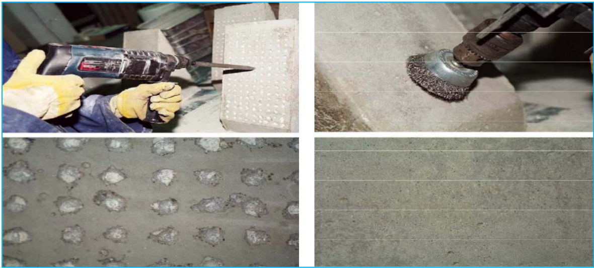
Figure I.10. A) Substrate surface partially chipped, B) Substrate surface prepared with steel brush[14].
