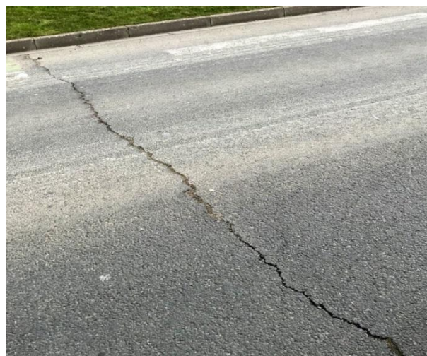
Figure II. 8 - Fissures transversales
