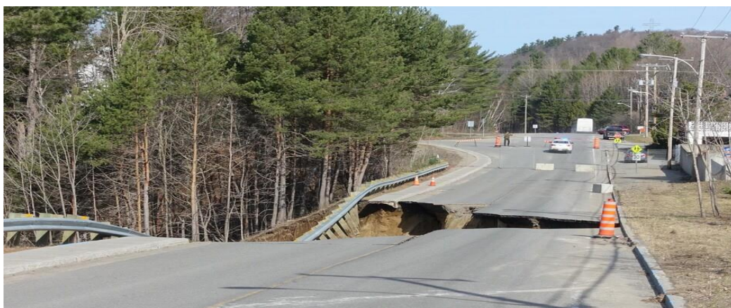
Figure II. 1 - Affaissement
