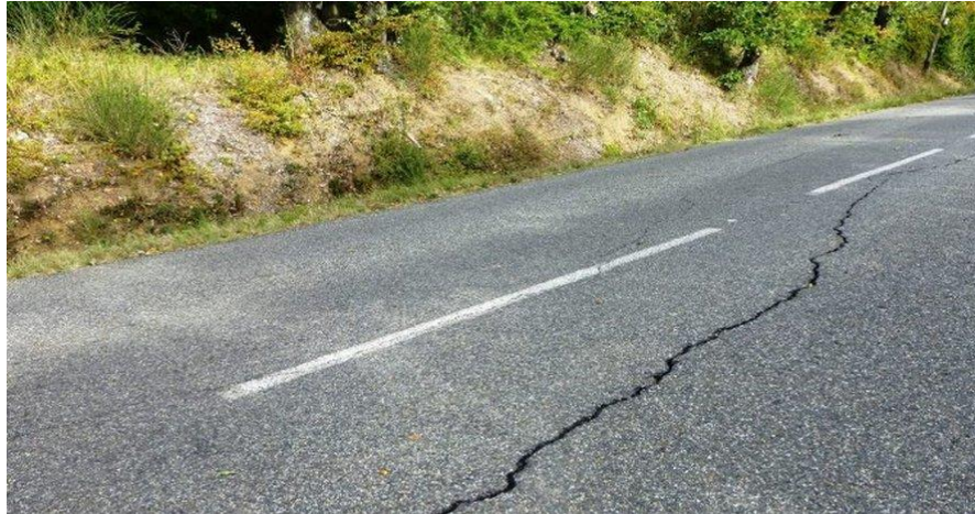
Figure II. 3 - Fissures de fatigue
