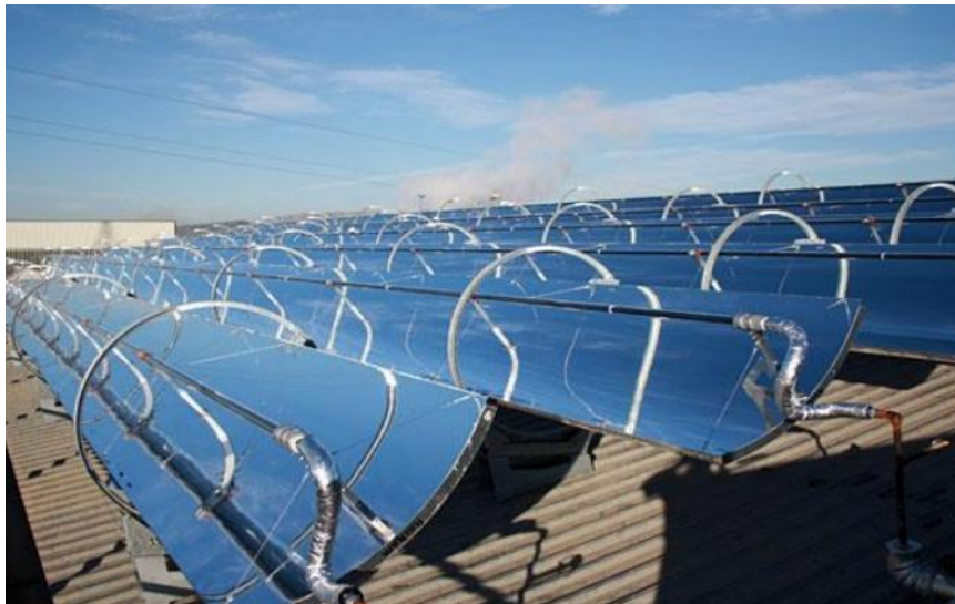
Fig 23: Cylindrical-parabolic solar power plant [42].
