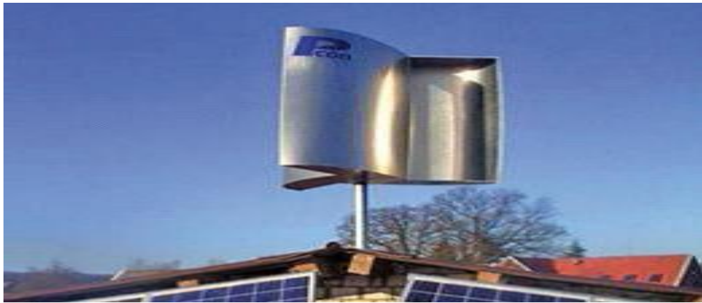
Fig 10: Savonius type wind turbine [9].
