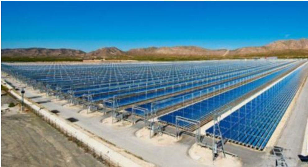
Fig 24: Solar power plant with Fresnel mirrors [42].
