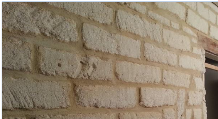
Figure II.20: mortier de chaux source : http://www.renov-it.com/wp-content/uploads/2013/10/mur_a_la_chaux.jpg
