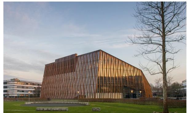
Figure 70 : Energy Academy Europe Source: ArchDaily
