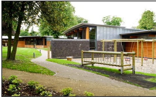
Figure 6: Utilisation de matériaux naturels, Hazel Wood School Source : http://www.topboxdesign.com
