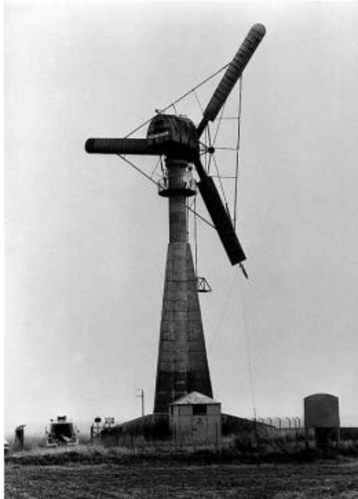
Figure I- 7 : Gedser wind turbine, 200 kW, D = 24 m, Denmark 1957[6].
