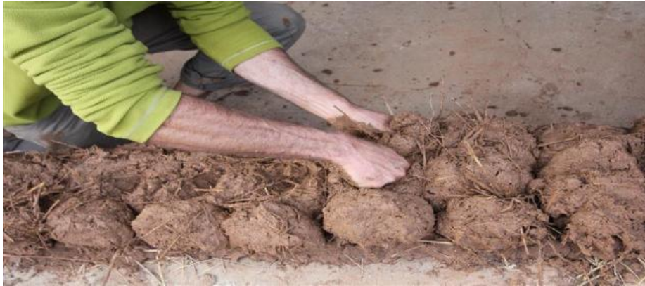
Figure I.11: la bauge
